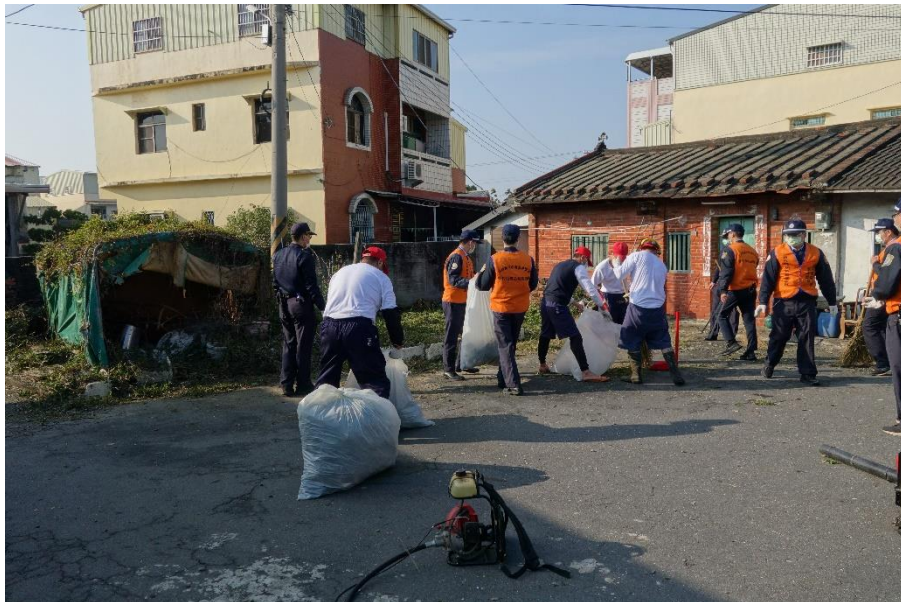
Actual cleaning execution (2)
