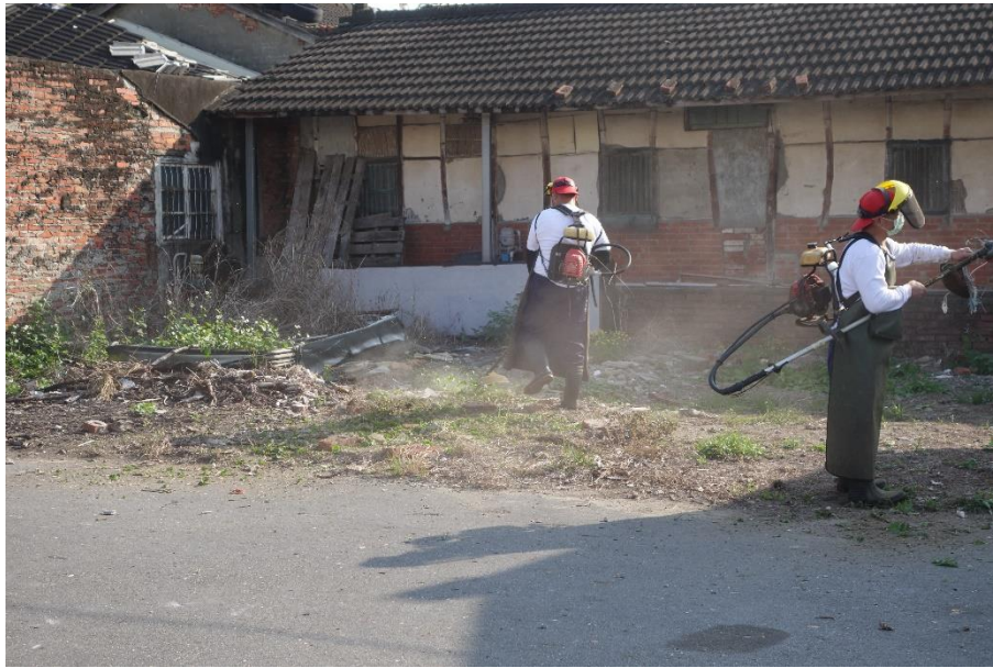
Actual cleaning execution (3)
