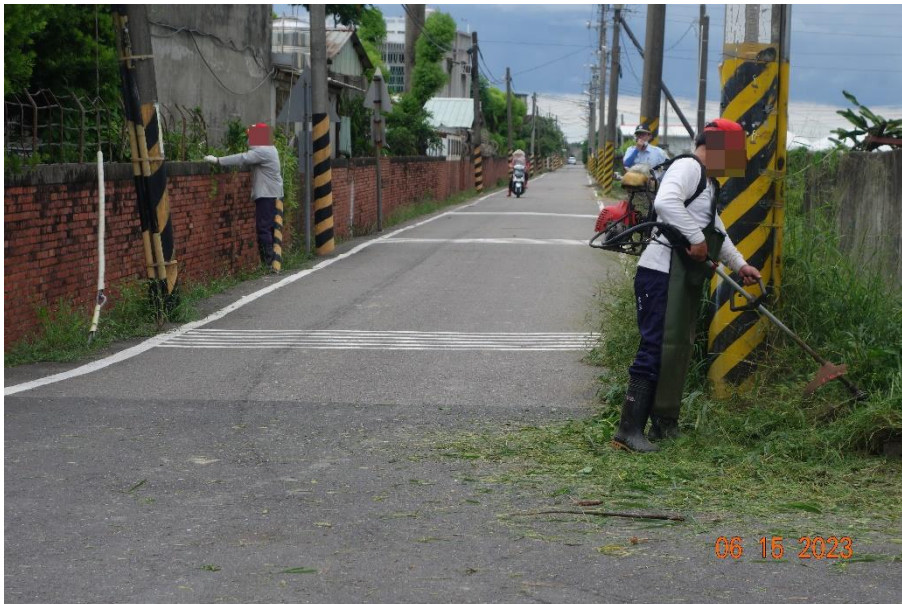
Actual cleaning execution (1)
