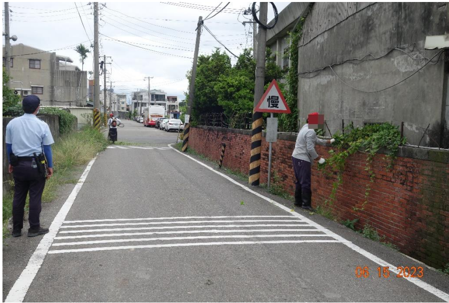
Actual cleaning execution (2)
