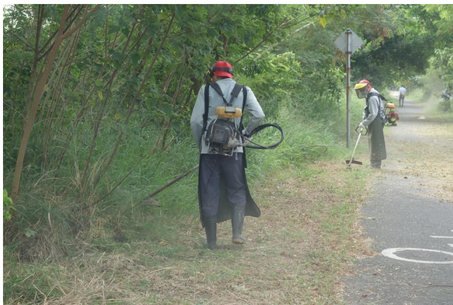
Actual cleaning execution (3)
